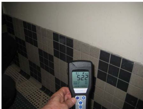
10.1 Hallway Floor Men's Area
